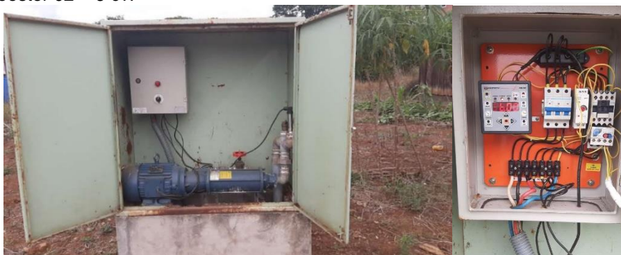
Figura 44: Booster 02 – 6 cv.
